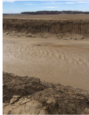
Picture # 7 – Dredged ditch w/o erosion control after a heavy rain.
