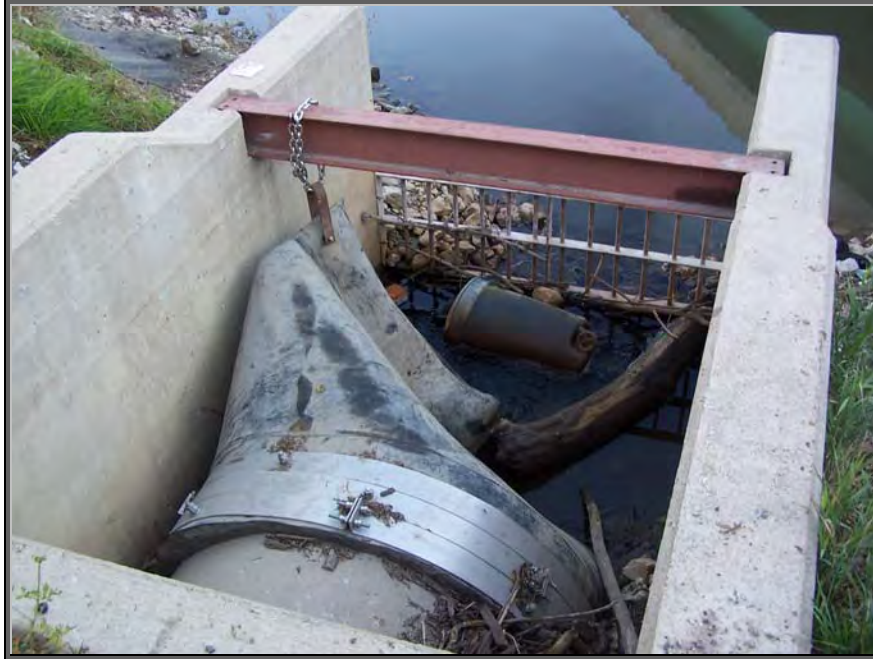
Figure 10 (SRS Location 6): Degraded storm outfall structure into the Little Calumet River. The bank at this location also seems to be eroding.
