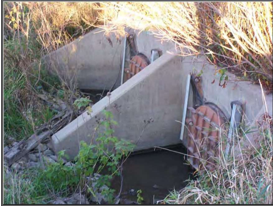
Figure 4 (SRS Location 2): Combined spill overflow structures at sampling location 38 that drain directly into the Little Calumet River without any type of treatment.
