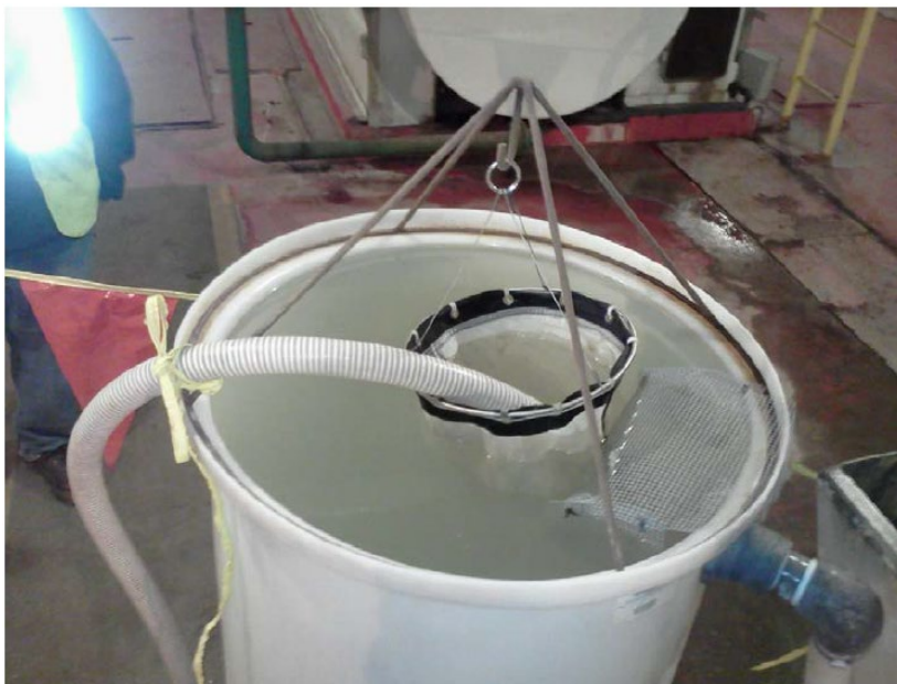
Photo 2. Holding Tank and Plankton Net at Lakeside Pump Station
