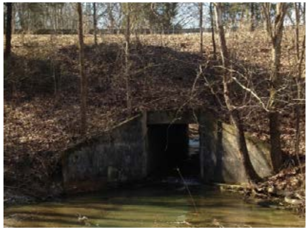
Figure 1-13 Windshield Site 936 - Tower Ridge Road at Combs Branch. Perched culvert.
