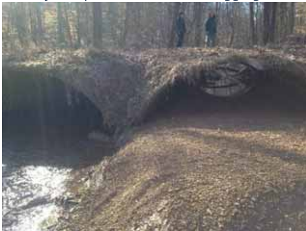
Figure 1-13 Windshield Site 936 - Tower Ridge Road at Combs Branch. Perched culvert.
