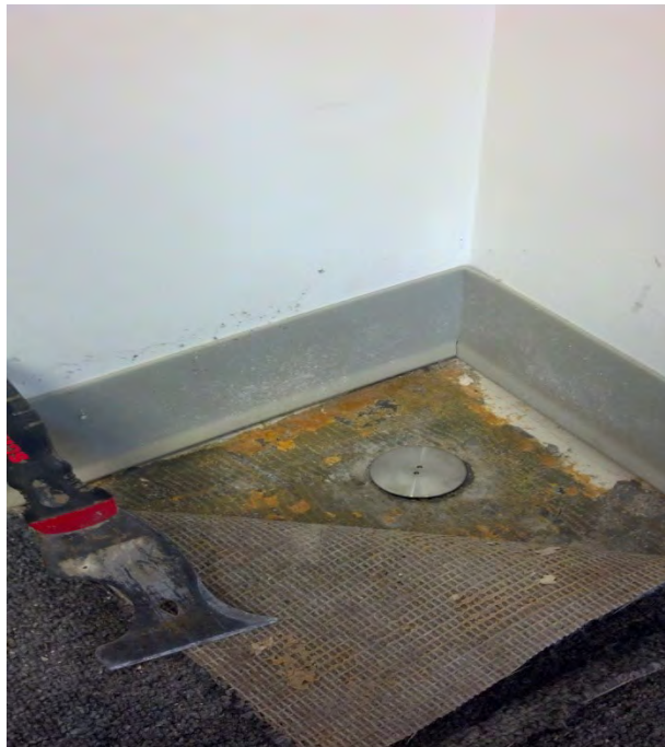
Protectant flush mounted cover over the Vapor Pin™
