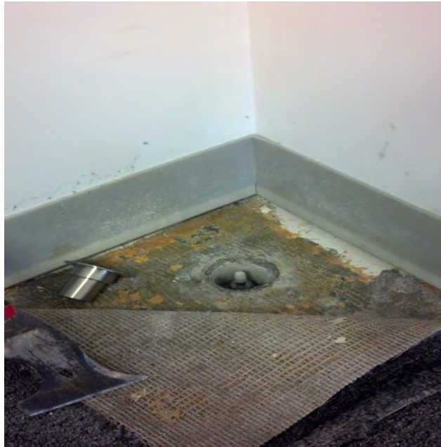
Final subslab installation appears of the Vapor Pin™
