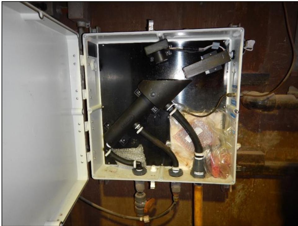
Photograph 10. No. 4 Steel Plant Treatment System – View of the turbidimeter for Outfall 618.
