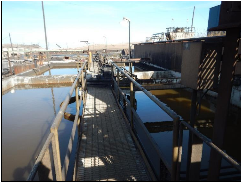
Photograph 27. No. 7 Blast Furnace Blowdown Treatment System – View, facing east, of the plant's two clarifiers.
