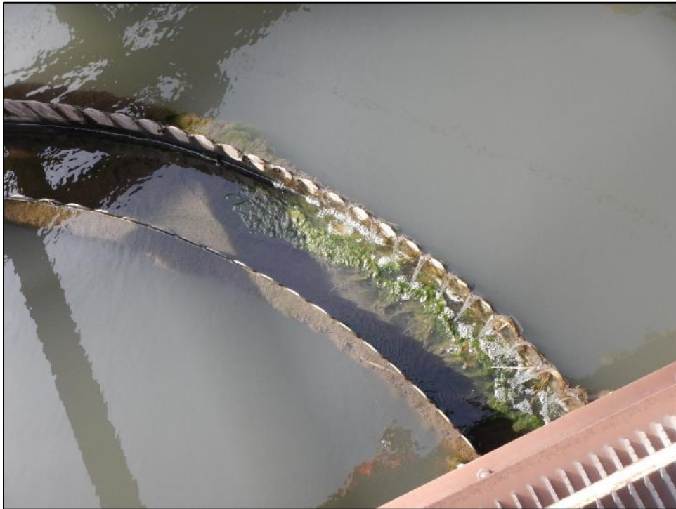
Photograph 36. No. 3 Sewage Treatment Plant – View of algae in the weirs of the secondary clarifier.
