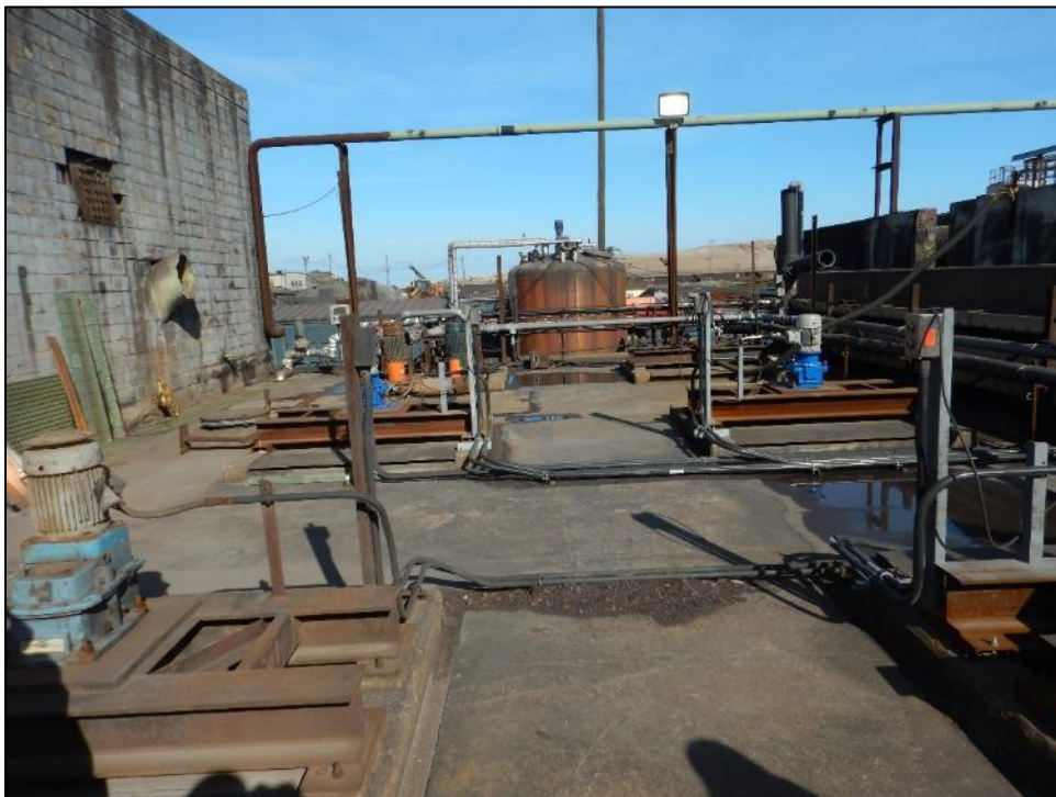
Photograph 28. No. 7 Blast Furnace Blowdown Treatment System – View, facing east, of the plant's multiple reaction chambers.
