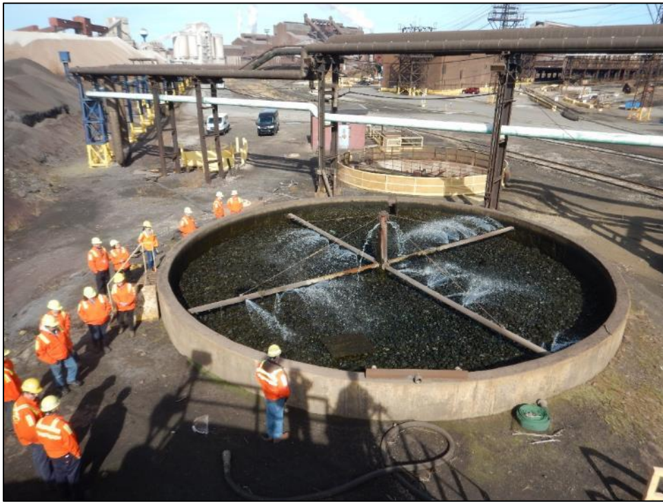
Photograph 35. No. 3 Sewage Treatment Plant – View of the trickling filter.
