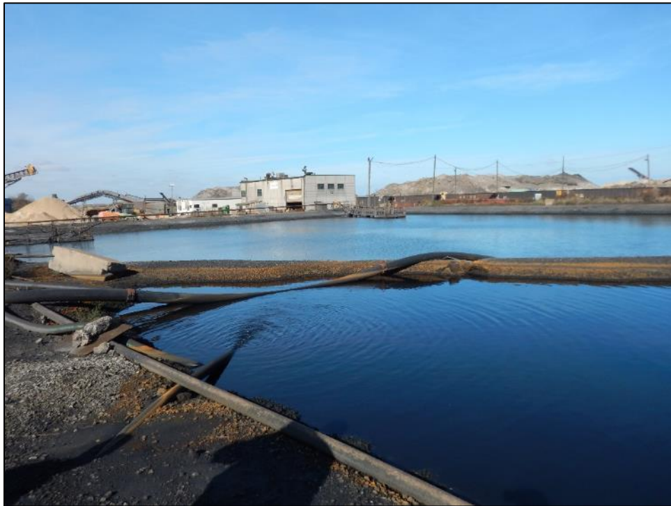
Photograph 24. No. 7 Blast Furnace Blowdown Treatment System - View, facing northeast, of the process wastewater ponds. The small pond section in the foreground of the photo feeds the treatment system.
