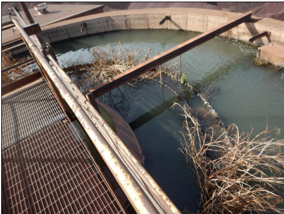
Photograph 34. No. 3 Sewage Treatment Plant – View of vegetation in the primary clarifier weirs.
