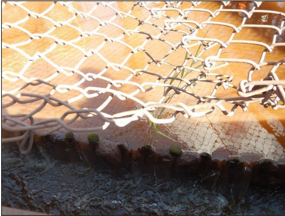
Photograph 7. No. 4 Steel Plant Treatment System – View of vegetation and algae in the north clarifier weirs.
