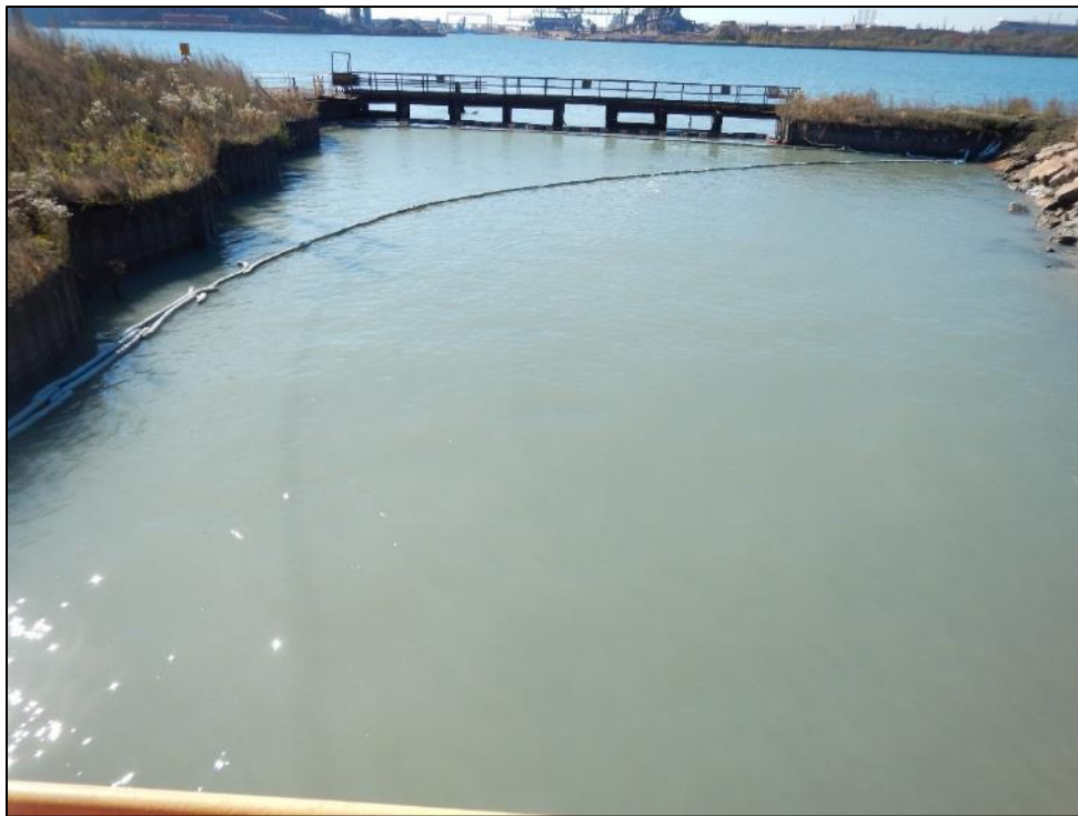
Photograph 2. Outfall 018 – View, facing west, of the Outfall 018 discharge area. Note the water was cloudy. Facility representatives stated they believed the cloudy conditions were caused by recent precipitation and wind in the lake.
