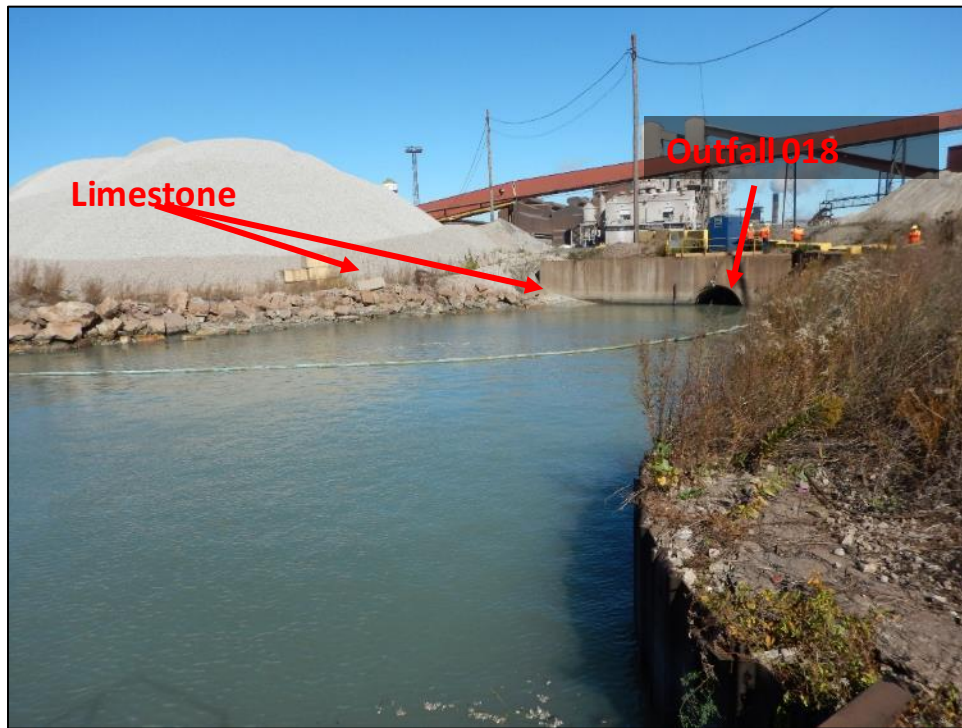
Photograph 5. Outfall 018 – View, facing north, of Outfall 018 and adjacent limestone stockpile. Note that the material was stored beyond the concrete barrier containment and some material had migrated to the edge of the receiving water.
