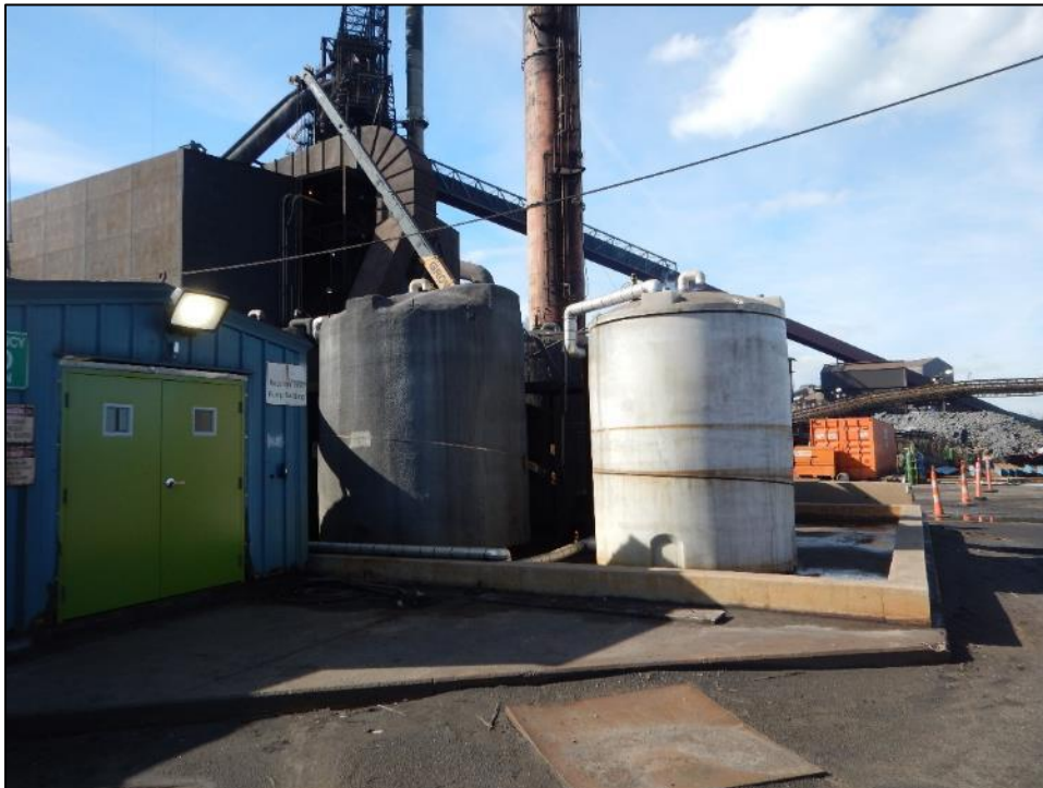
Photograph 26. No. 7 Blast Furnace Blowdown Treatment System – View, facing north, of sulfuric acid and ferric chloride chemical and mixing tanks.
