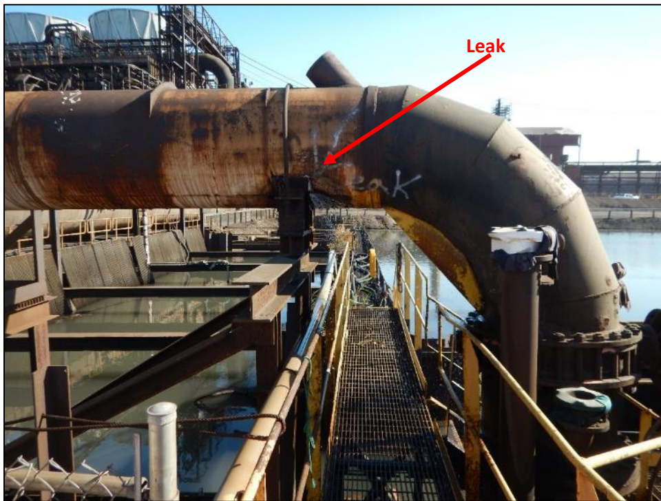
Photograph 14. Terminal Treatment Plant West - View of a leak in a pipe entering the effluent channel.
