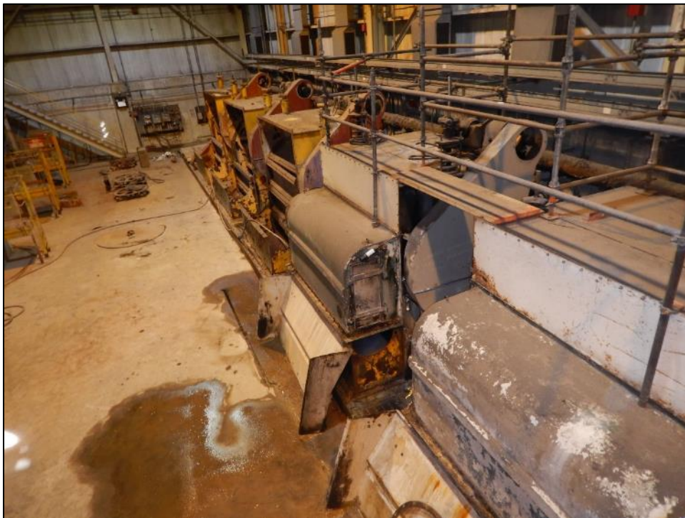
Photograph 32. No. 7 Pump House – View of the intake screens inside the pump house building.
