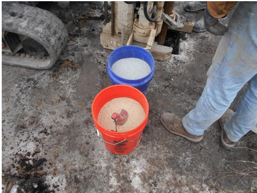
4. View of filler sand and bentonite chips used at each well location
