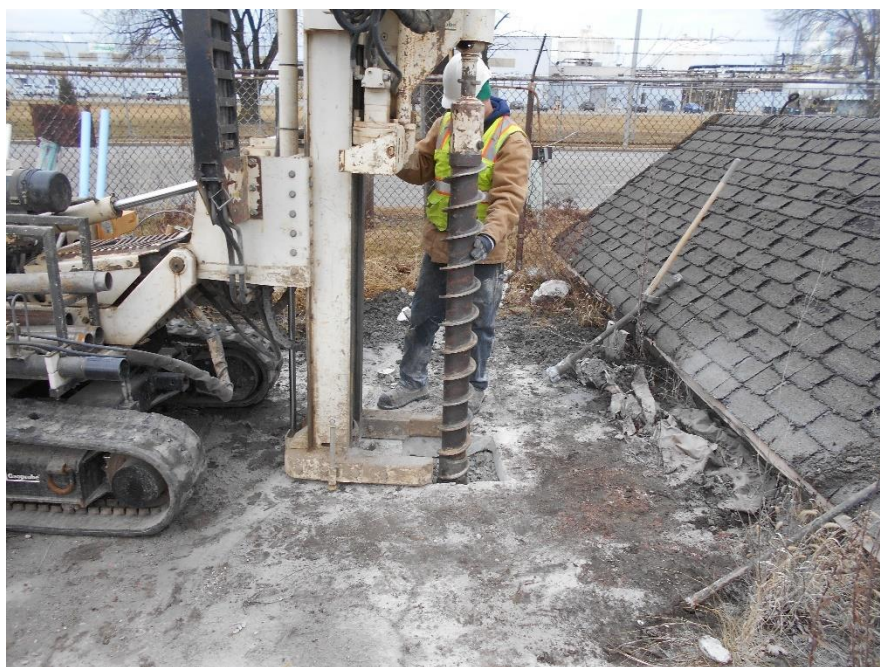
1. Shallow augering at MW-1
