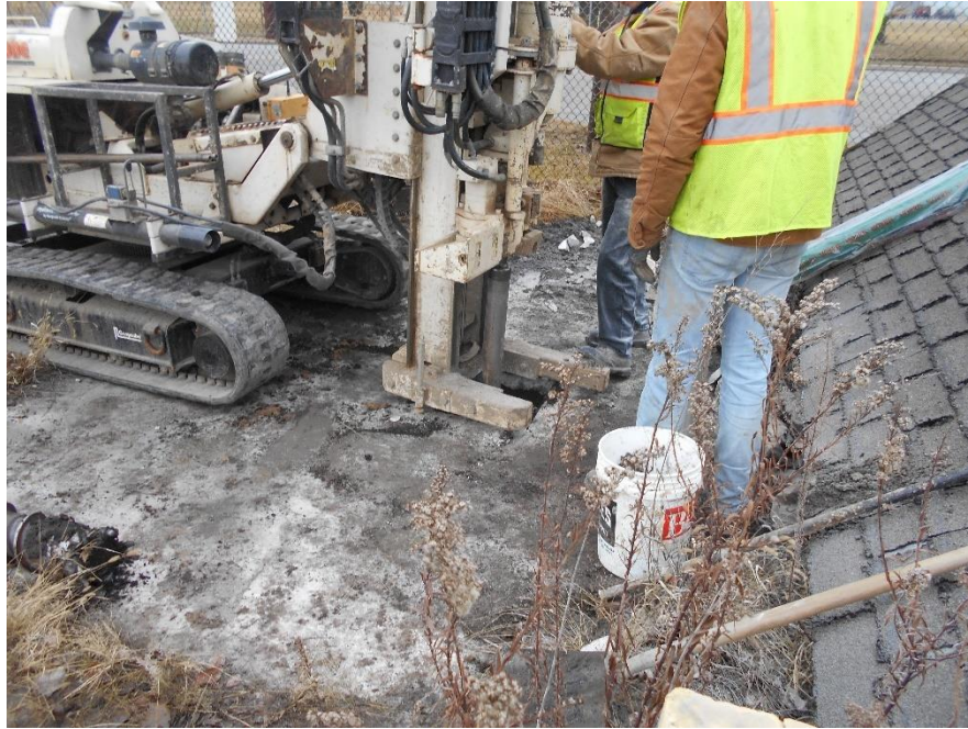
3. View of well advancement at MW-1
