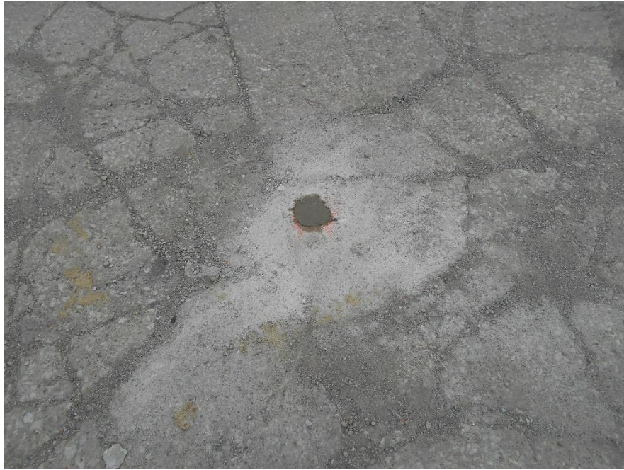
37. Typical probe hole surface repair
